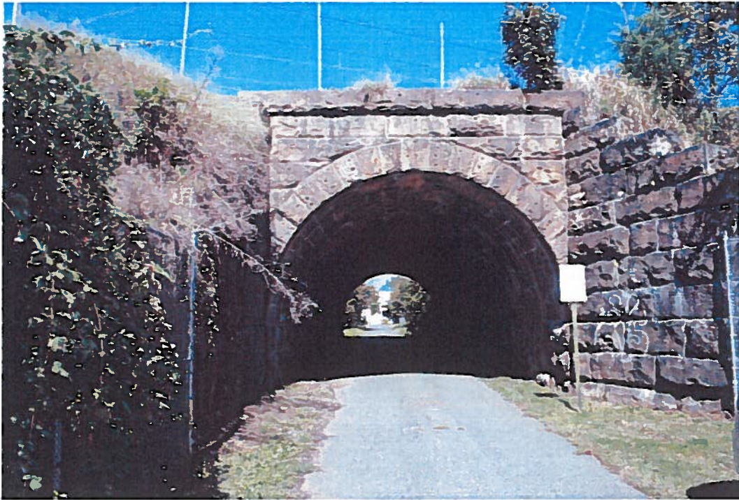
South entrance to Centennial Lane overpass
