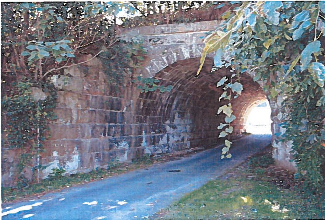
North entrance to Freedom overpass
