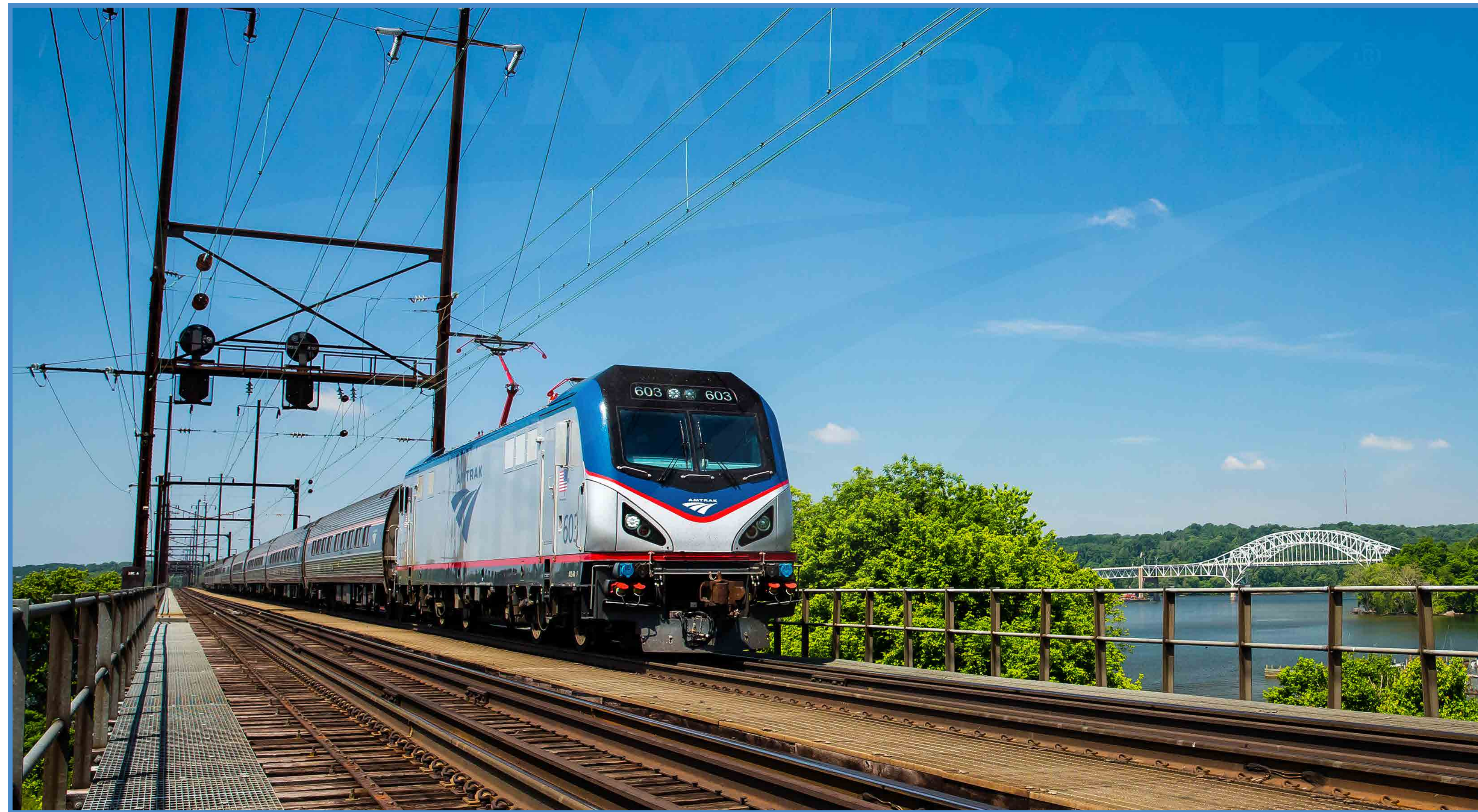
Amtrak train crossing the Susquehanna River Rail Bridge
