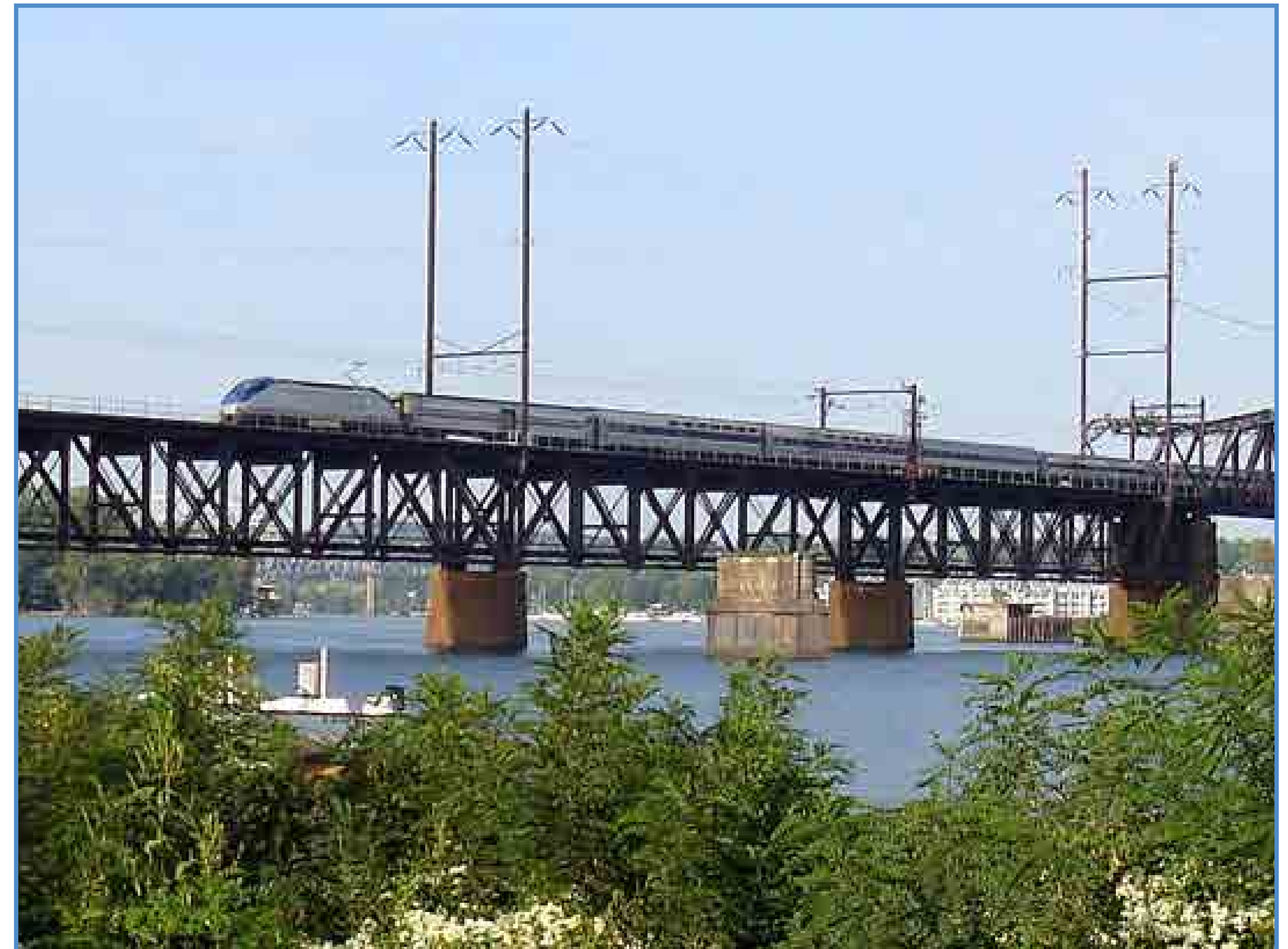
Amtrak train crossing the Susquehanna River Rail Bridge
