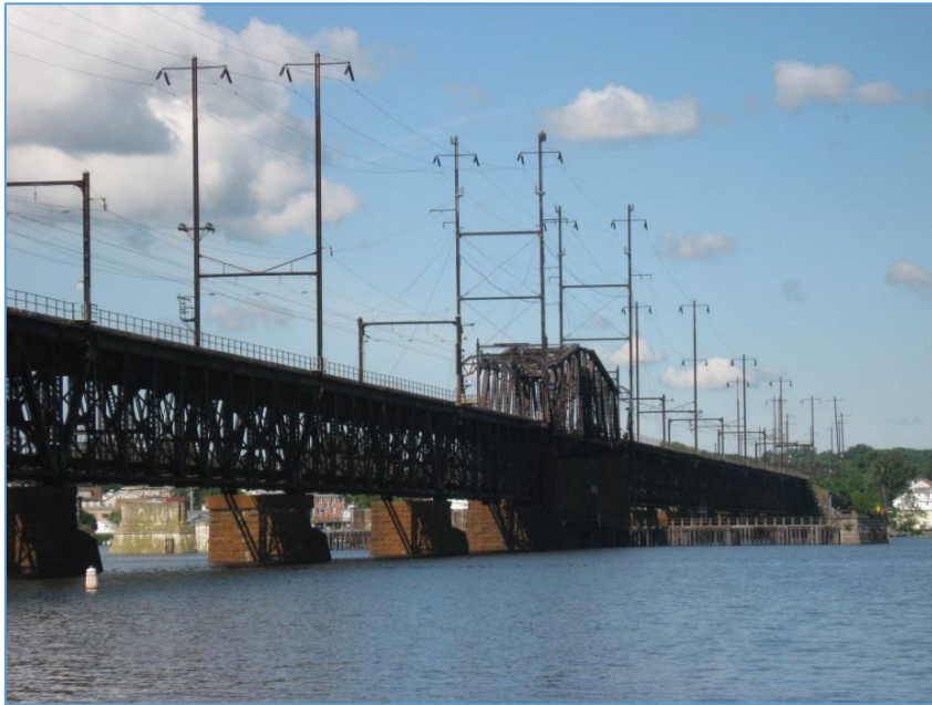
Amtrak Railroad Bridge over the Susquehanna River
