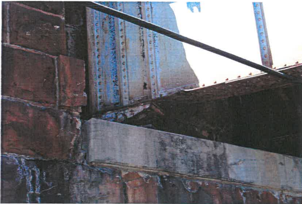
Abutment chop-out & capping at Juniata Street
