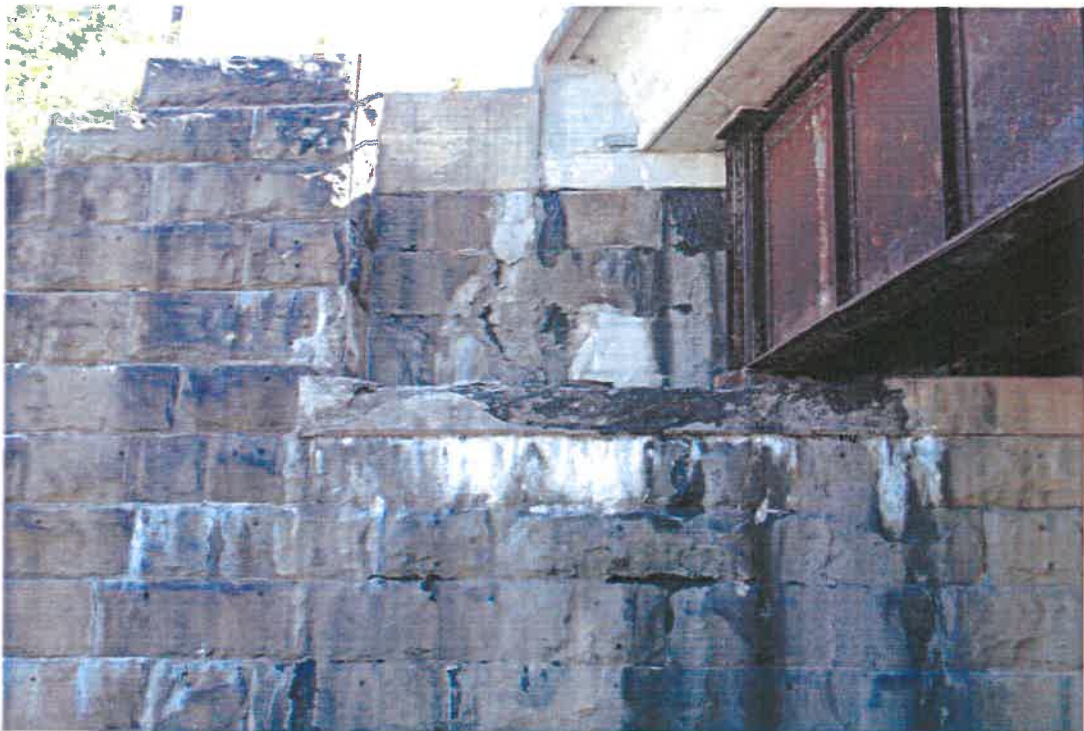
Chop-down, chop-out, concrete caps, plate girder modification, leaching & discoloration at Stokes abutment
