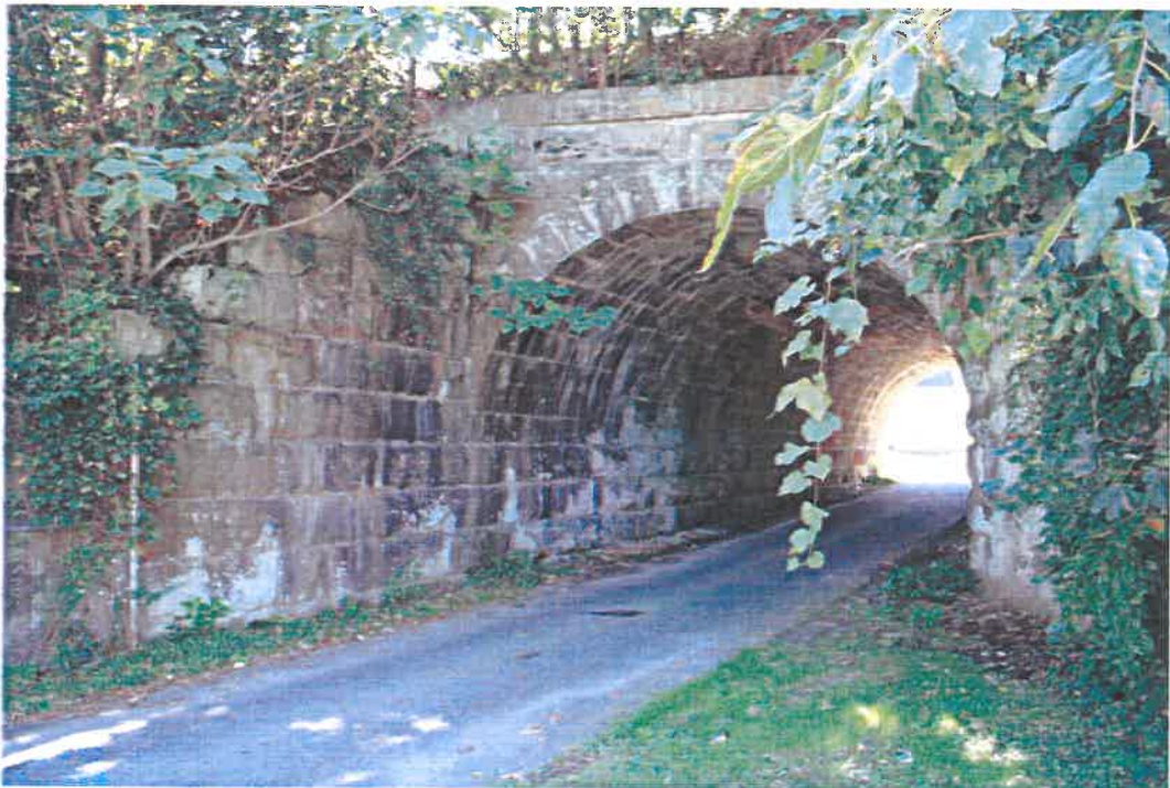
North entrance to Freedom overpass
