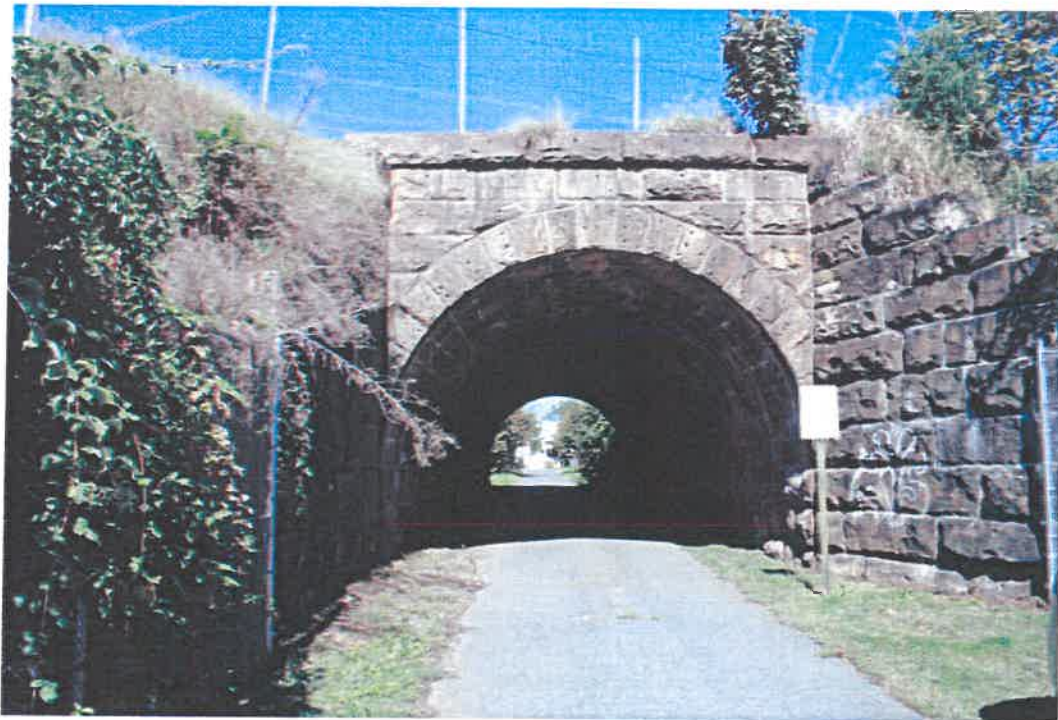
South entrance to Centennial Lane overpass
