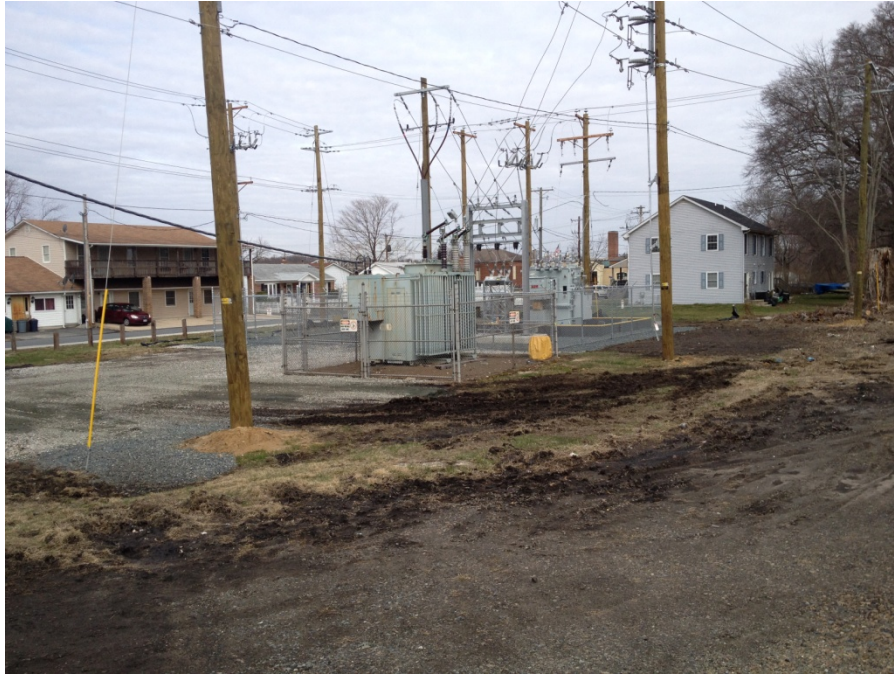
Norfolk Southern Railroad site, view to the northwest from Otsego Street.
