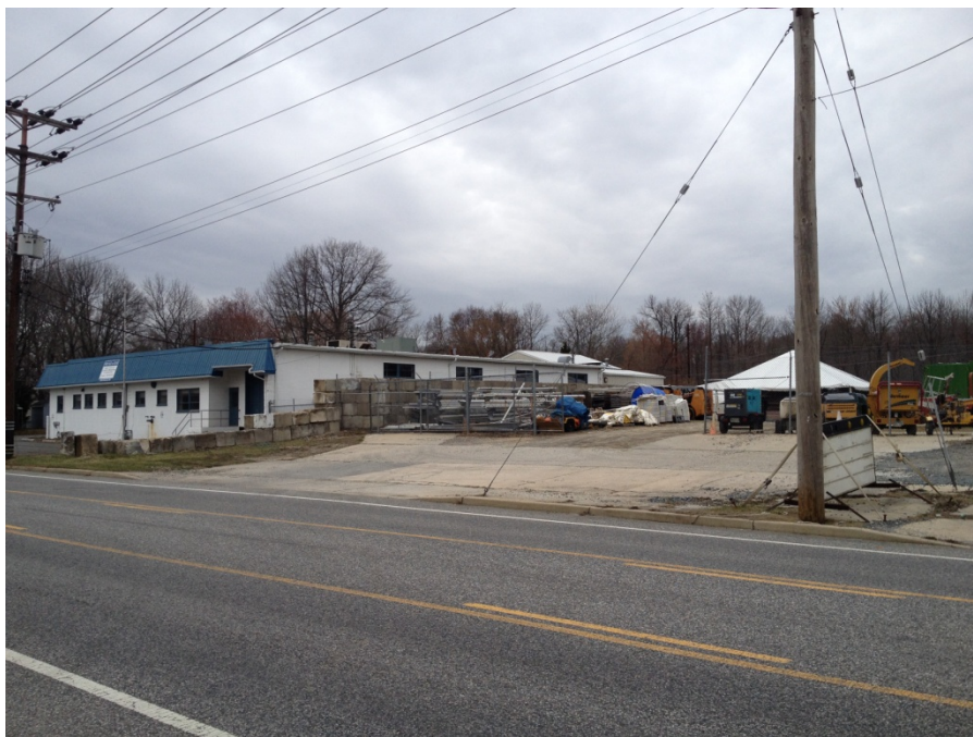
Former C&P Telephone site, view to the northwest.
