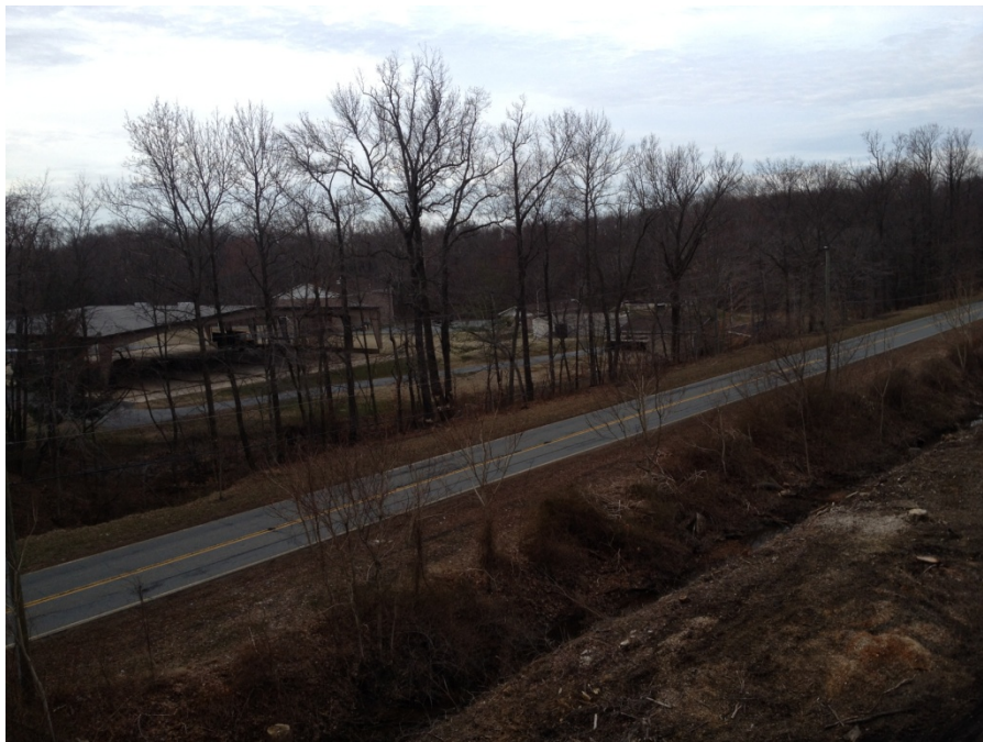
Perryville wastewater treatment plant, view to the southwest from Firestone Road bridge.
