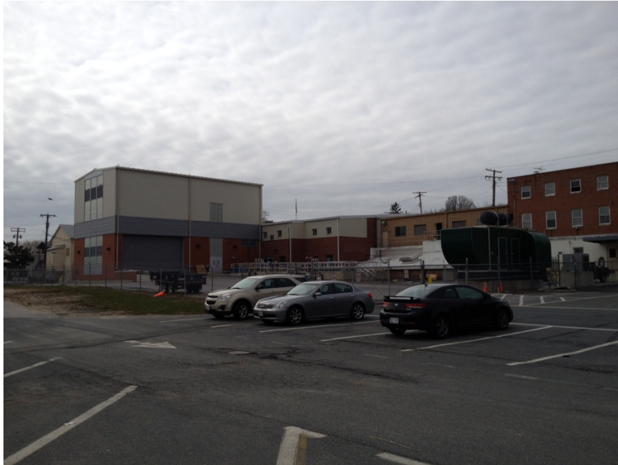
The HdG WWTP site, view to the southwest.
