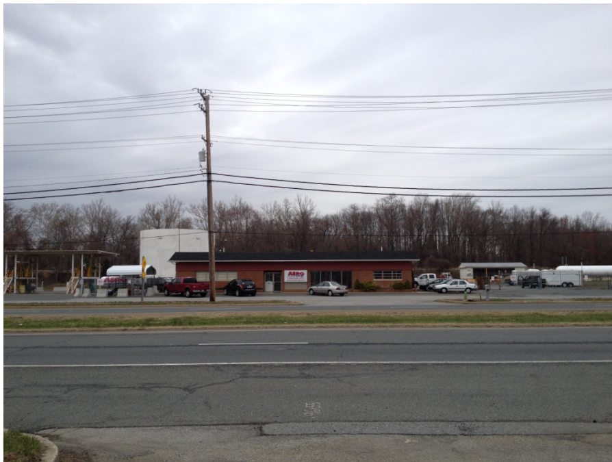
Aero Energy, view to the northwest from Pulaski Highway.
