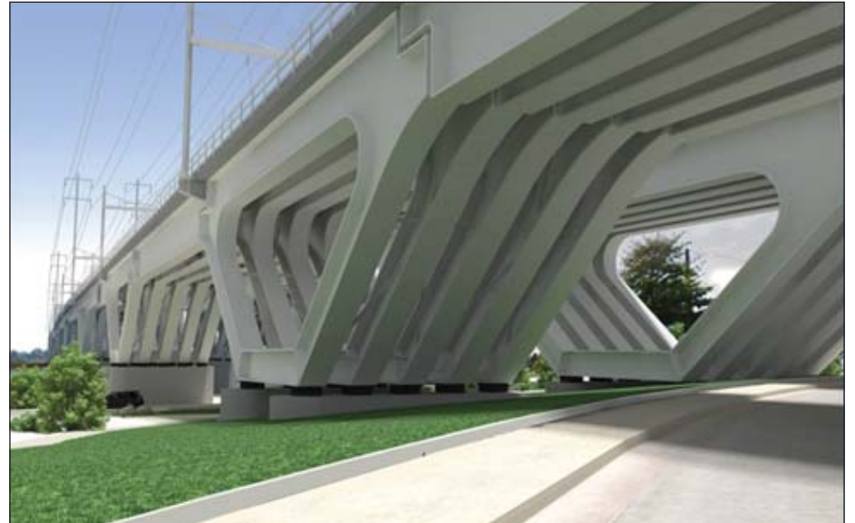
Delta Frame Pier Design
