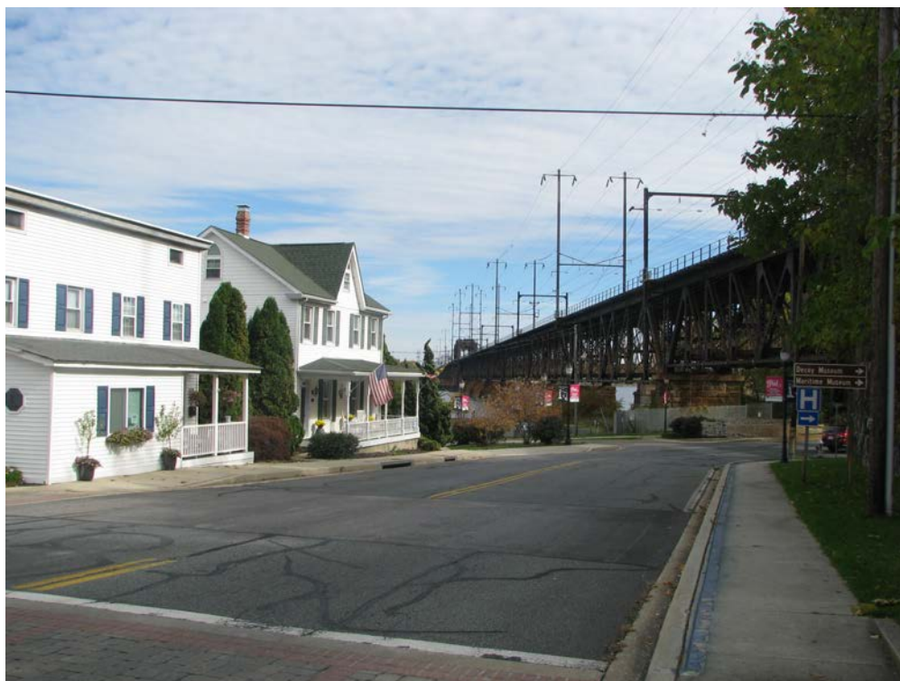
Otsego / Water Streets: late nineteenth / early twentieth century houses; looking east. 10
