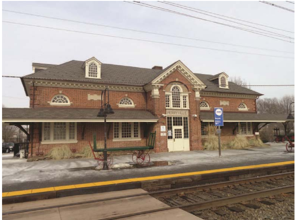
Perryville Railroad Station: view of the south elevation; looking north. 21
