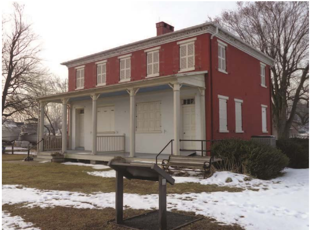
Toll House: View of the northeast and northwest elevations; looking south. 16
