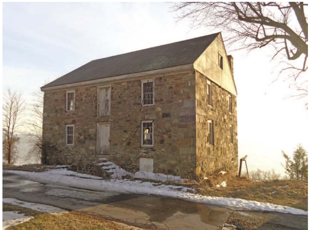
Perry Point Mill: view of the east façade; looking west. 20
