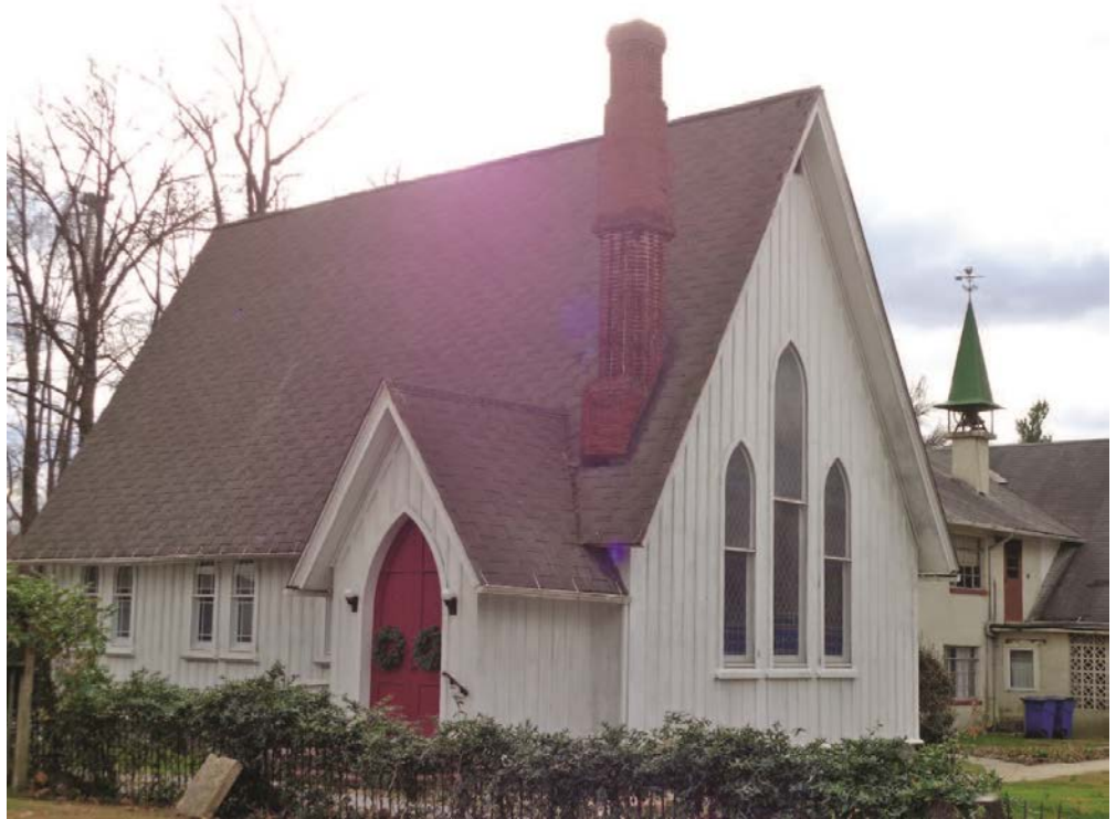
Perryville Presbyterian Church: view of the side (east) and front (north) elevations of the church at 710 Broad Street in Perryville; looking southwest. 31
