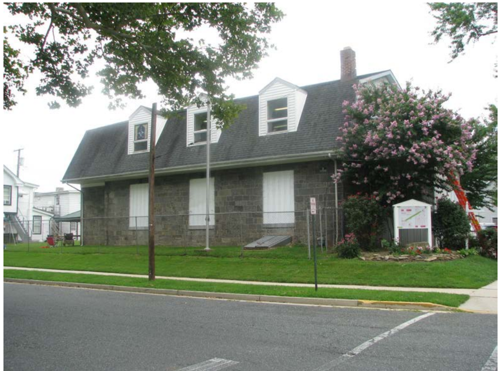
429 N. Stokes Street: Room at the Cross Mission Church (former St. Patrick's Catholic Church); looking southeast. 4
