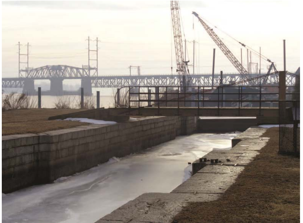
South Lock #1 and Toll House: Susquehanna Terminus, Susquehanna and Tidewater Canal; looking southeast. 15
