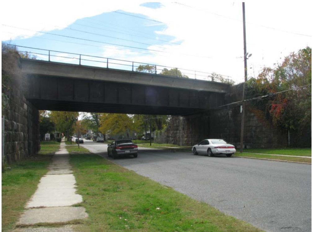
North Stokes Street Undergrade Bridge (MP 60.56): view of the railroad west side, 12 which will be altered via removing a portion of the existing stone masonry abutment and building a new concrete abutment; looking south.
