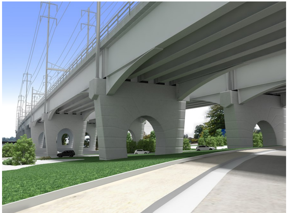
Rendering of possible arched piers to be used with the girder approach; looking east from Havre de Grace. 37
