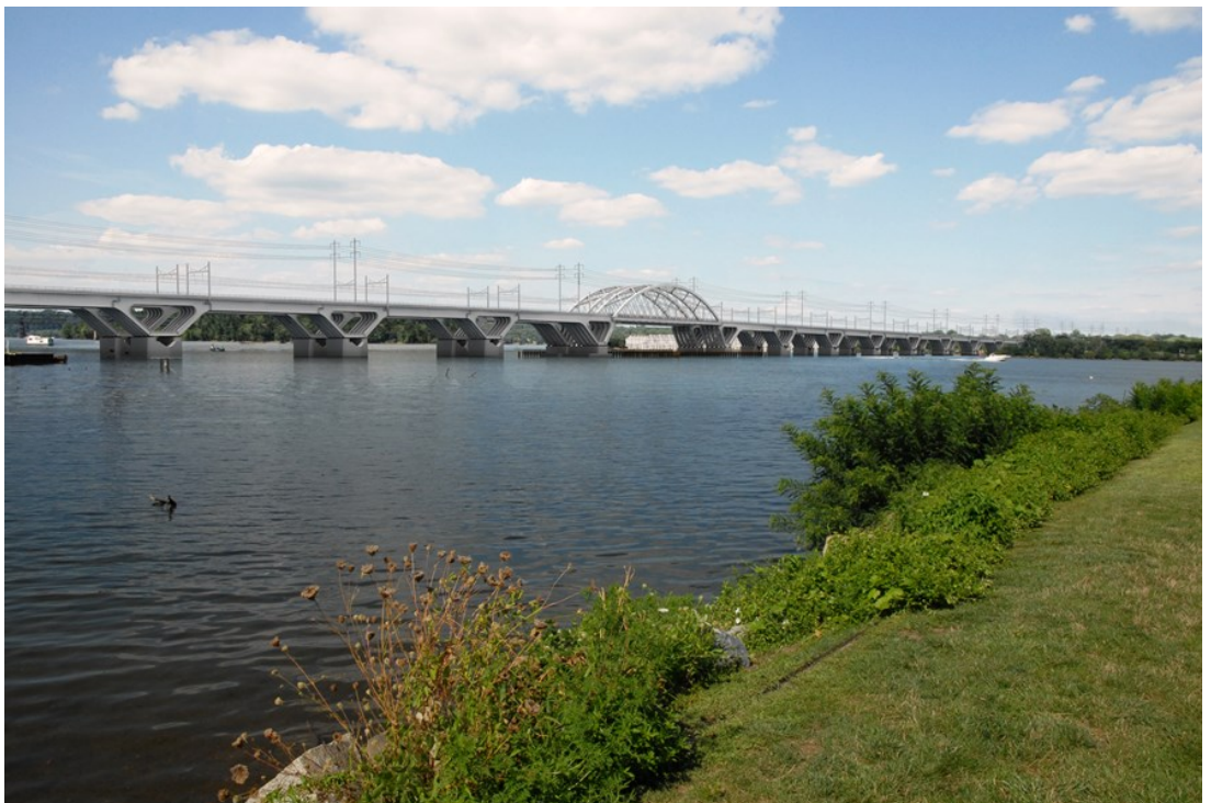
Rendering of a proposed replacement bridge with a Delta frame approach and arch main span; 35 looking northeast from Havre de Grace.
