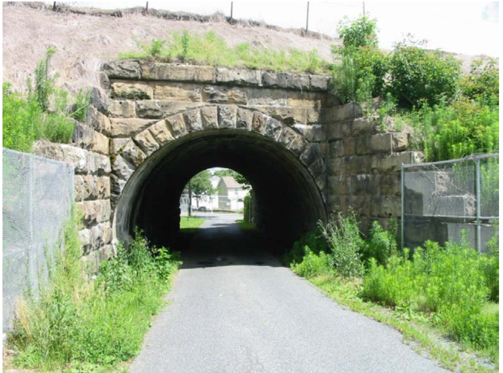
North Freedom Lane Undergrade Bridge (MP 60.51): view of the railroad east side, 11 which will be altered via removing the existing stone-arch culvert and replacing it with a precast concrete culvert; looking north.
