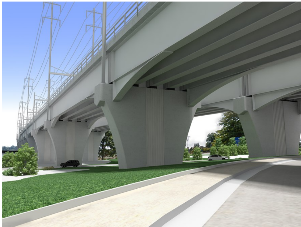
Rendering of possible fluted piers to be used with the girder approach; 38 looking east from Havre de Grace.
