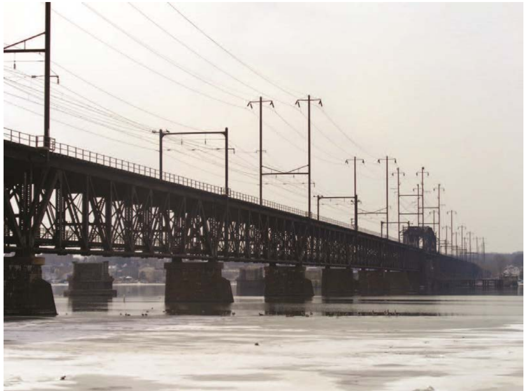
Susquehanna River Rail Bridge: View from the Perryville waterfront; looking southwest.
