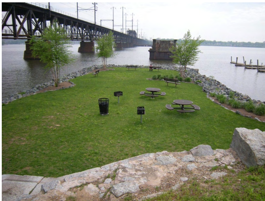
Photograph 23: View of David Craig Park (Study Area 3), facing east-northeast. Note PW&B abutment in foreground.
