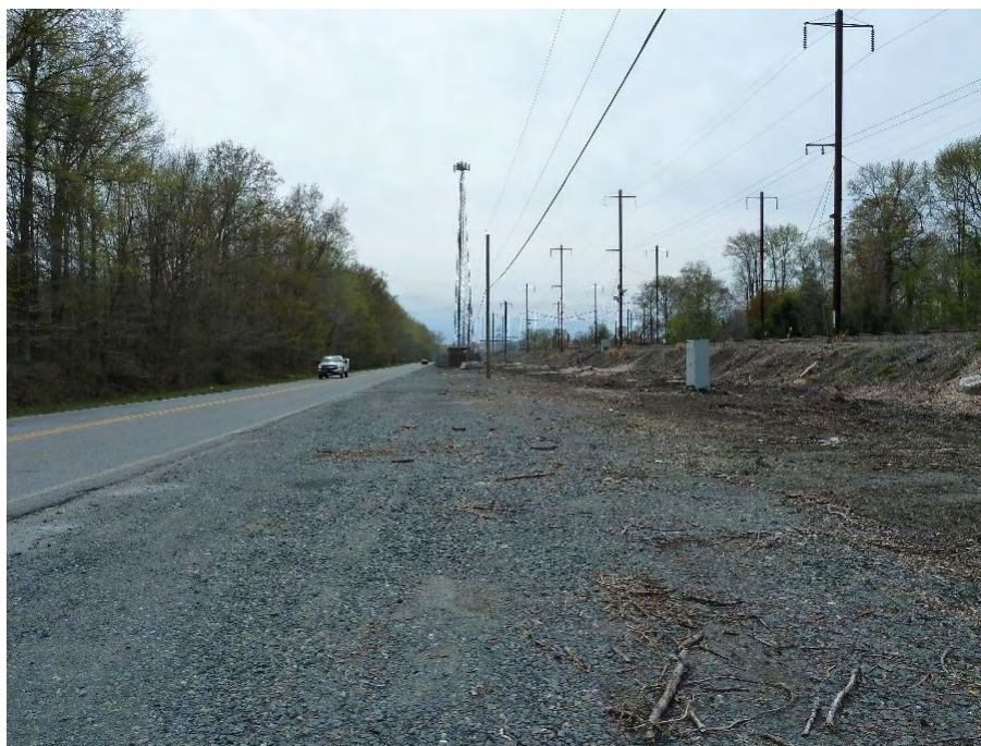
Photograph 11: General view of disturbed Amtrak ROW along access road west of Avenue G, facing west.
