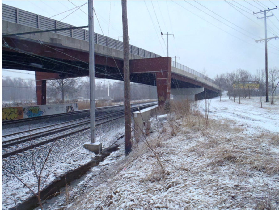
Photograph 7: General view of disturbed Amtrak ROW east of Revolution Street, facing west.
