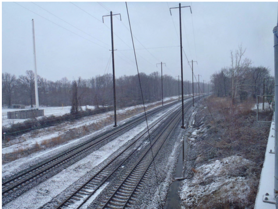
Photograph 8: General view of disturbed Amtrak ROW west of Revolution Street, facing west.
