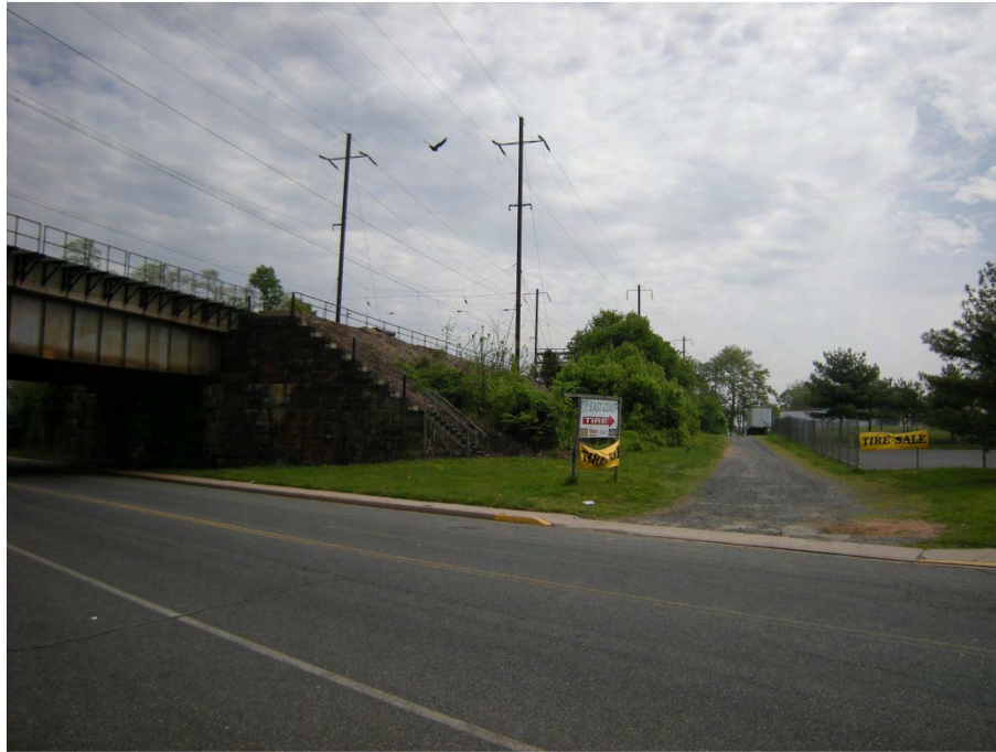
Photograph 19: Representative view of rail corridor along Warren Street within Study Area 2, facing northeast.
