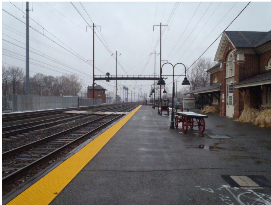
Photograph 10: General view of Perryville Station, facing west.
