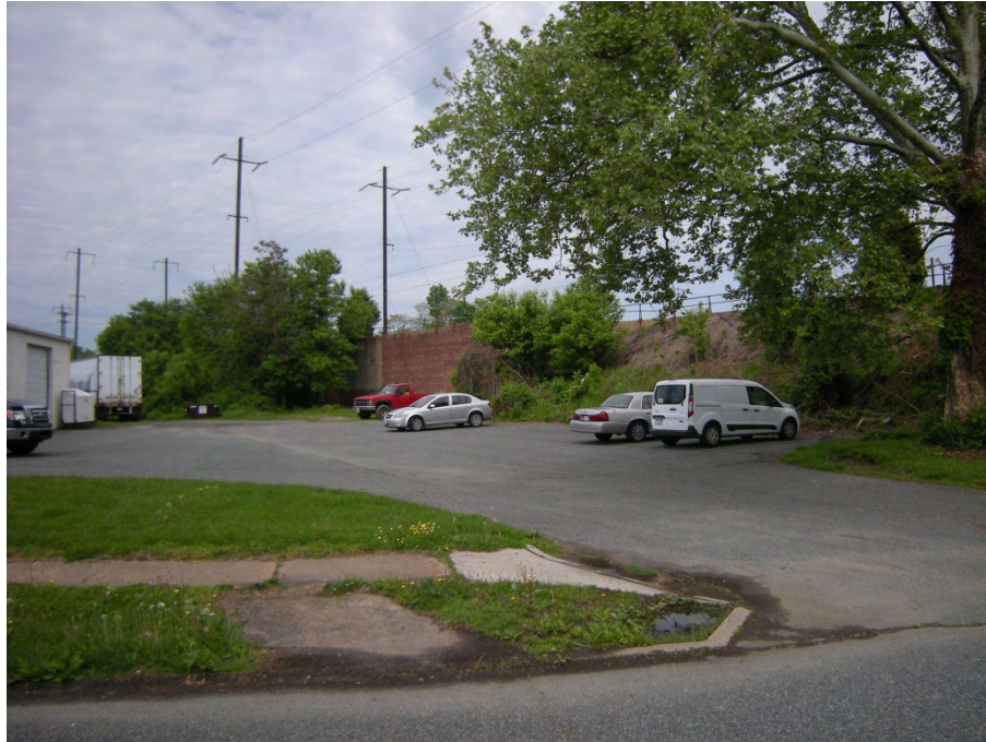
Photograph 21: View of potential remains of Havre de Grace train station within existing embankment, facing west.
