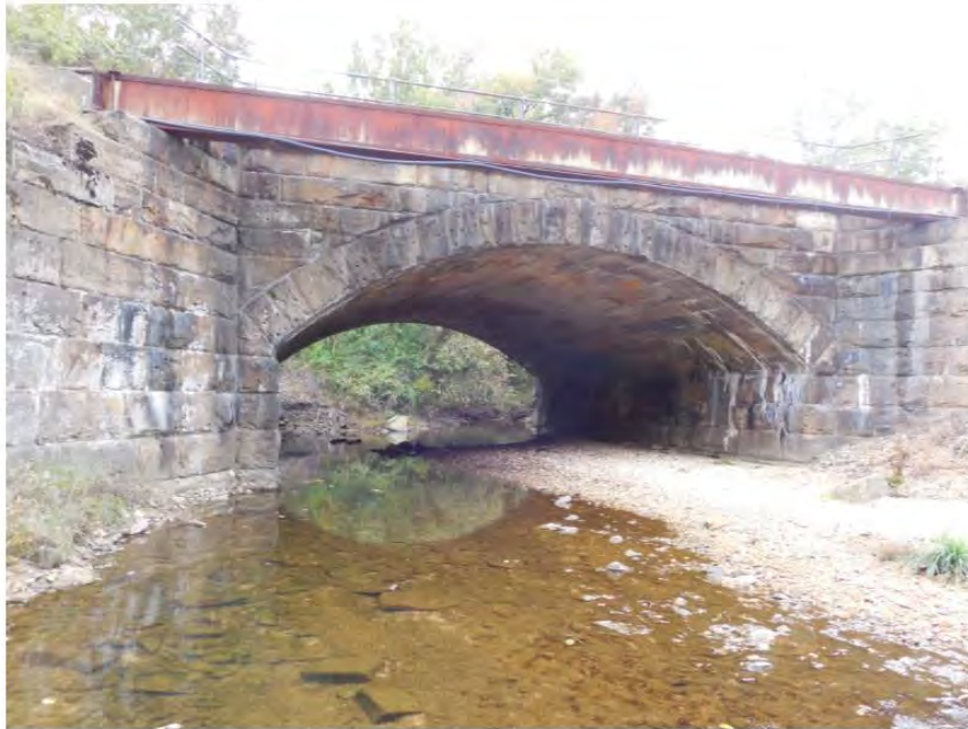
Photo 51: View looking northwest at the east side of the Mill Creek Undergrade Bridge (MP 59.00) that will be extended with a precast concrete culvert.
