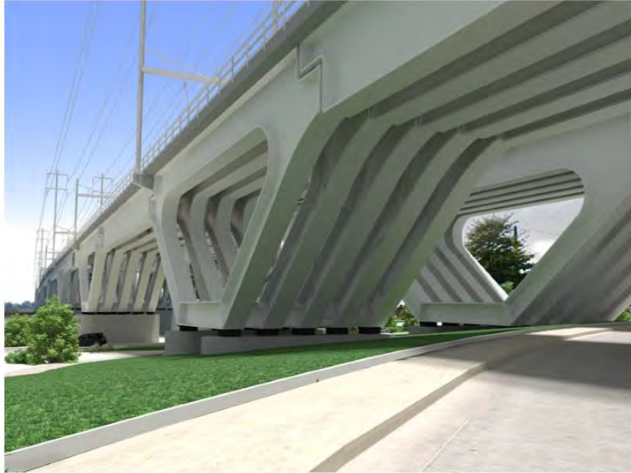
Photo 48: Rendering of the piers for the Delta frame approach. View looking east from Havre de Grace.
