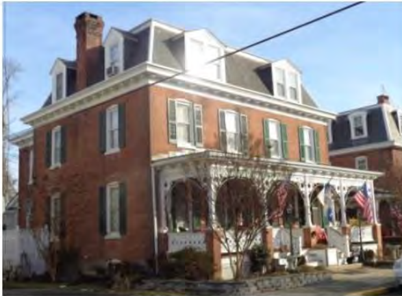
Photo 3: Representative mid-nineteenth century residential structure within the Havre de Grace Historic District.
