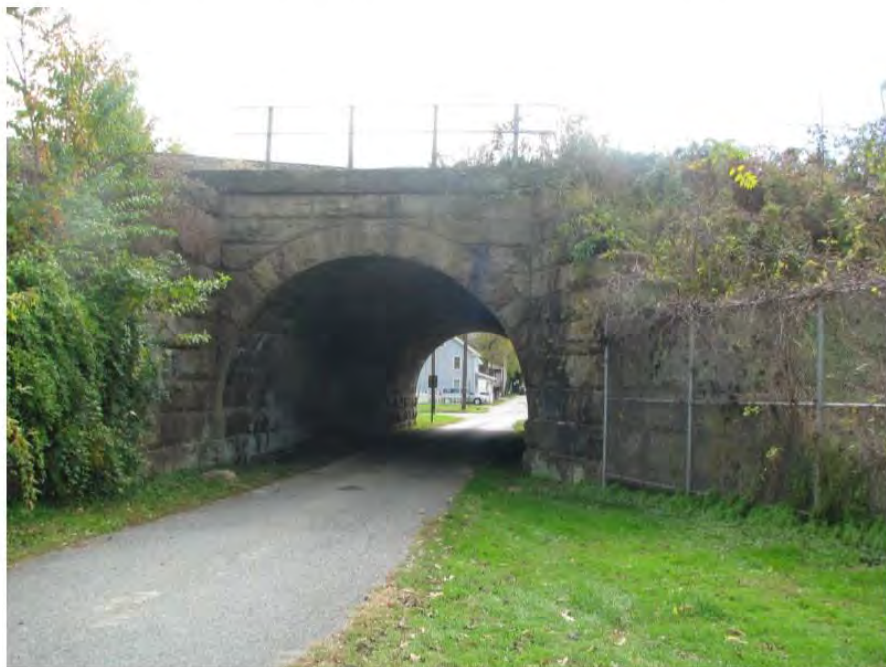
Photo 60: View looking south at the railroad west side of Centennial Lane Undergrade Bridge (MP 60.61), which will be extended with a precast concrete culvert.
