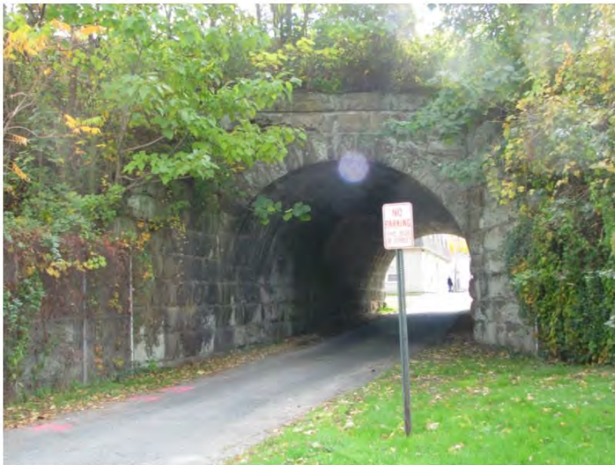
Photo 56: View looking south at the railroad west side of North Freedom Lane Undergrade Bridge (MP 60.51), which will be altered via construction of a precast concrete culvert.
