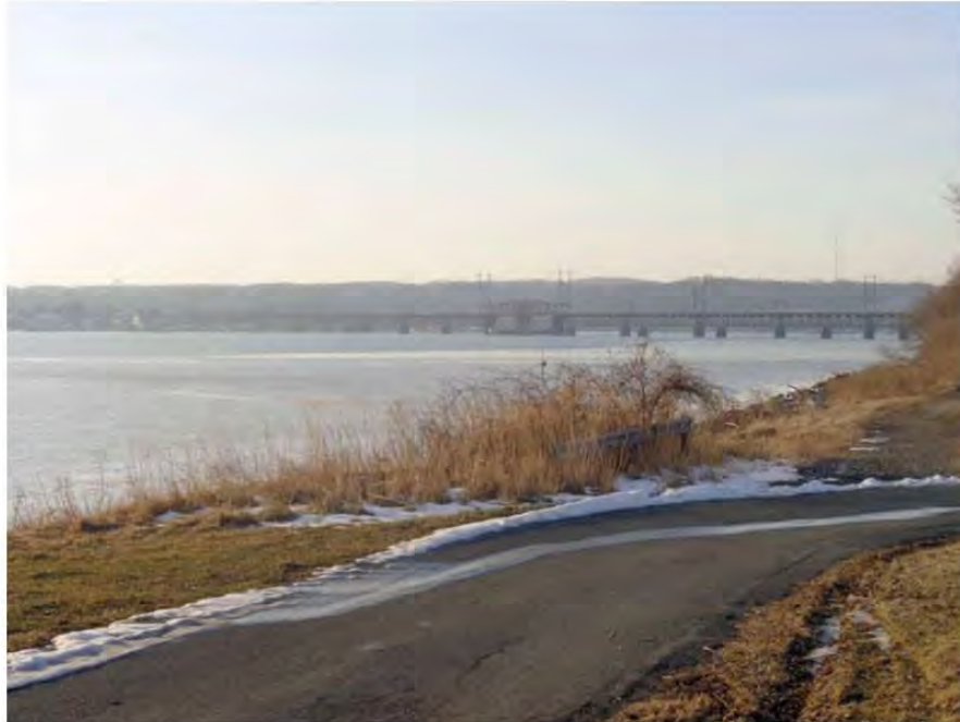
Photo 82: View looking northwest towards the Susquehanna River Rail Bridge from a waterfront walking path near the Perry Point Mansion and Mill.
