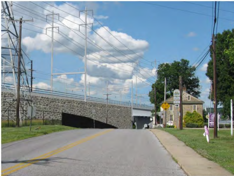
Photo 79: Rendering showing the proposed retaining wall to be constructed in front of Rodgers Tavern, with a possible aesthetic design solution.
