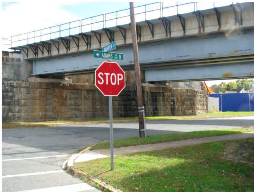
Photo 62: View looking southeast at the railroad west side of North Adams Street Undergrade Bridge (MP 60.69) that will be extended with a concrete abutment.
