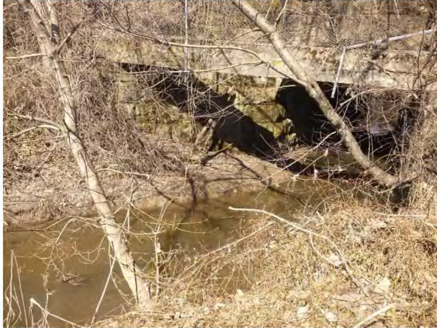
Photo 64: View looking northeast at the railroad east side Lily Run Undergrade Bridge (MP 60.85) which will be spanned over by a multi-girder bridge.
