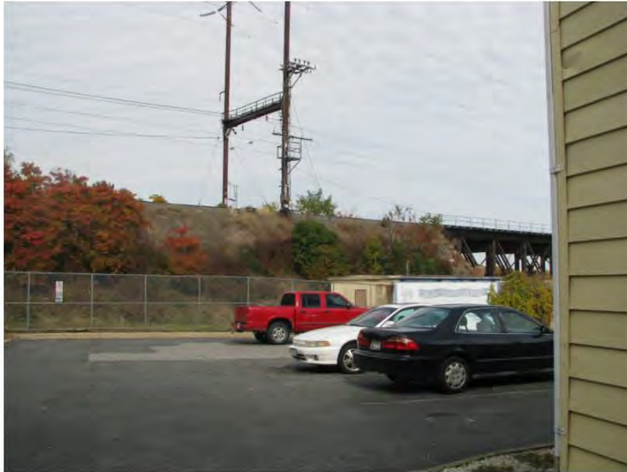
Photo 69: View looking north from the rear of 511 Warren Street, showing its current relationship to the railroad tracks. The setting of this house will be altered by the proposed widening that will bring the tracks either 13 feet closer (Alternative 9B) or 30 feet closer (Alternative 9A).
