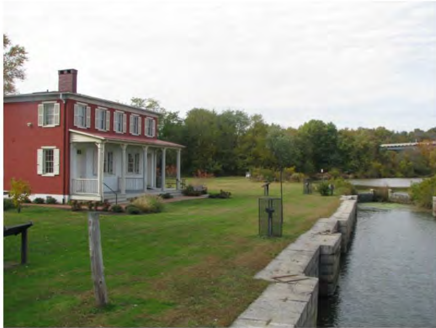
Photo 32: View looking north at the Southern Terminus, Susquehanna and Tidewater Canal- South Lock #1 and Toll House.
