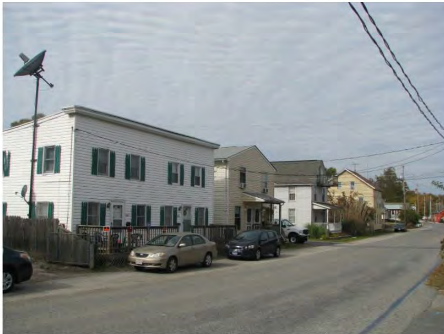
Photo 30: View looking northwest at nineteenth century structures along Water Street.
