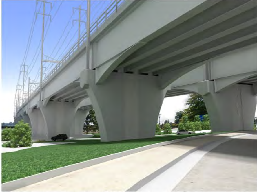
Photo 50: Rendering of possible fluted piers to be used with the girder approach. View looking east from Havre de Grace.
