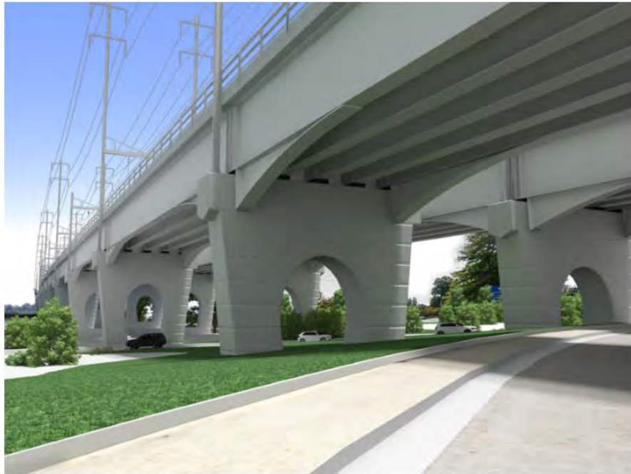
Photo 49: Rendering of possible arched piers to be used with the girder approach. View looking east from Havre de Grace.
