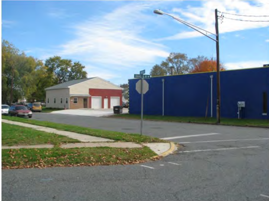
Photo 15: View looking southeast from the corner of N. Adams Street and Warren Street towards modern commercial structures along Warren Street.
