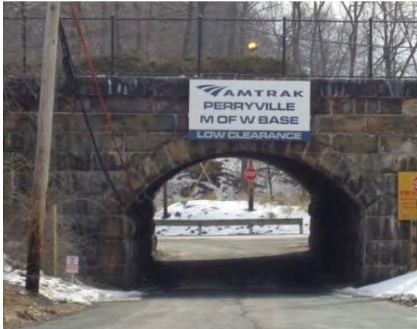
Photo 38: View looking south at the Perryville Railroad Station Undergrade Bridge.
