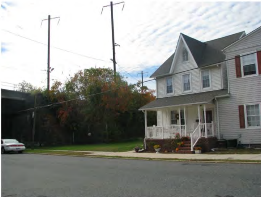
Photo 68: View looking southwest at the mid-nineteenth century house at 518 N. Stokes Street in relation to the railroad tracks. The setting of this house will be altered by the proposed widening that will bring the tracks 26-28 feet closer to it.
