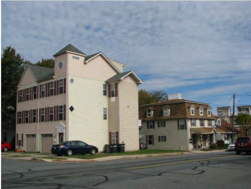
Photo 21: View looking northeast at the modern residential structure at the northeast corner of Otsego Street and N. Stokes Street.
