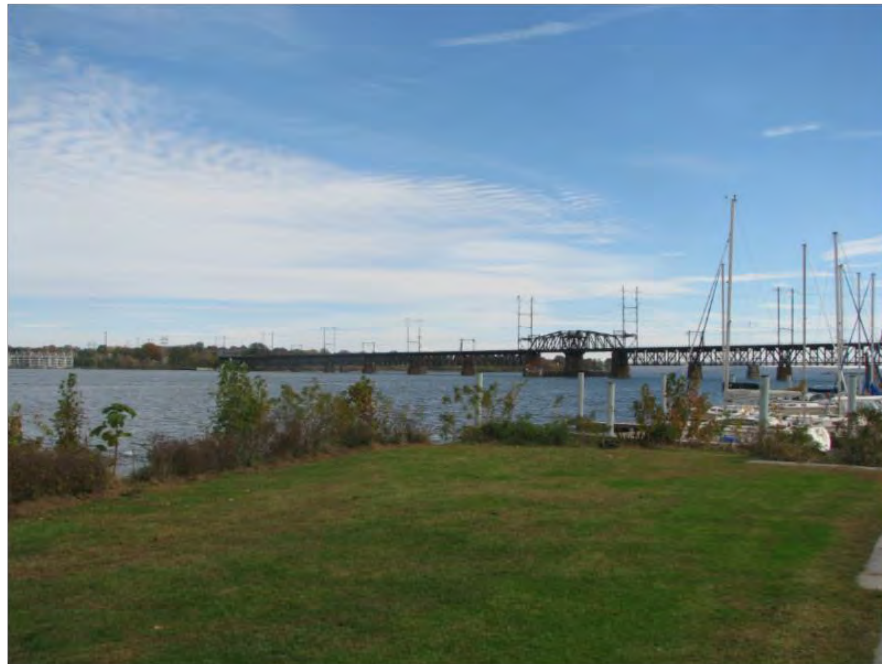
Photo 2: View looking southeast towards the Susquehanna River Rail Bridge from the Southern Terminus, Susquehanna and Tidewater Canal.
