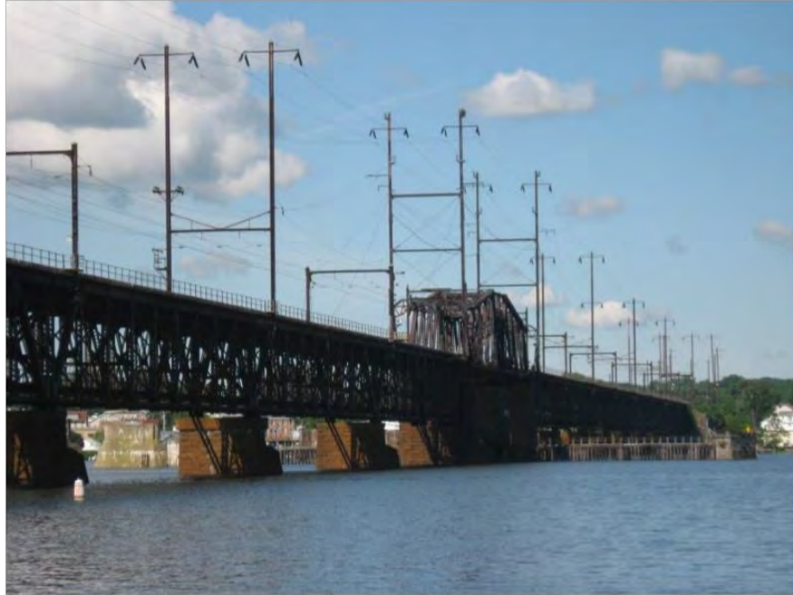
Photo 1: View looking southwest at the Susquehanna River Rail Bridge from Perryville.
