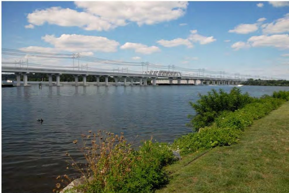
Photo 45: Rendering of a proposed replacement bridge with a girder approach and a truss main span. View looking northeast from Havre de Grace.
