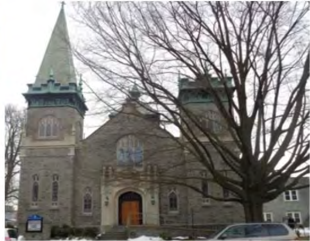
Photo 4: Representative masonry ecclesiastical structure within the Havre de Grace Historic District.
