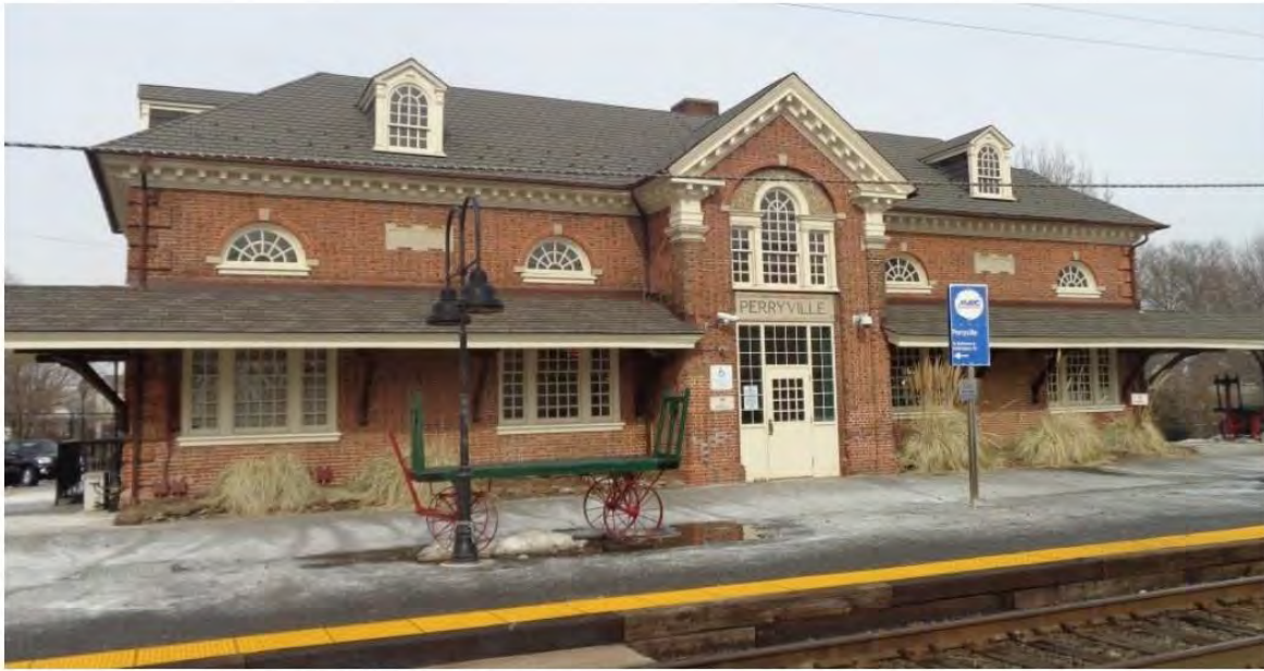
Photo 36: View looking northeast at the Perryville Railroad Station.
